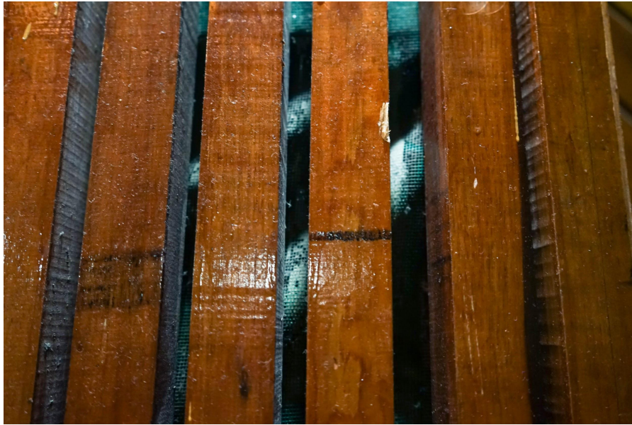
Wood wool board beneath vertical timber battens.
