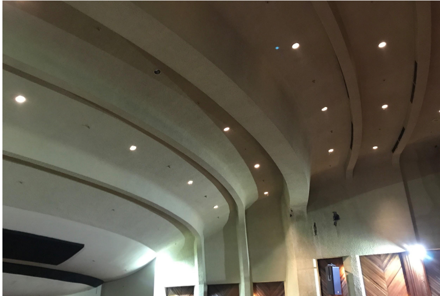
Smooth finish plaster ceiling of the whole auditorium.
