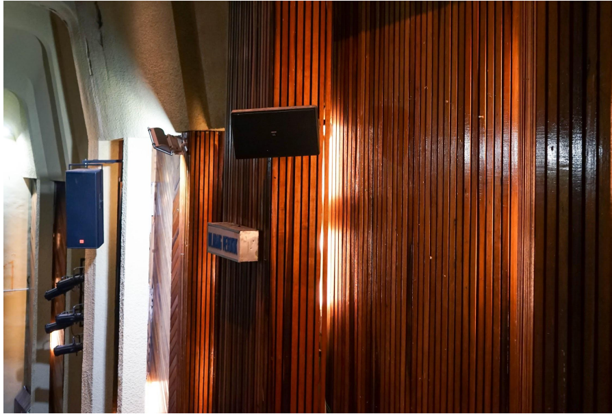
Vertical spaced timber battens on the side of the hall.
