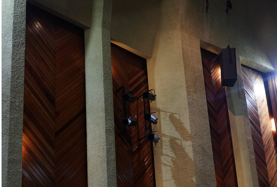
Rough concrete wall finish on the side of the hall.
